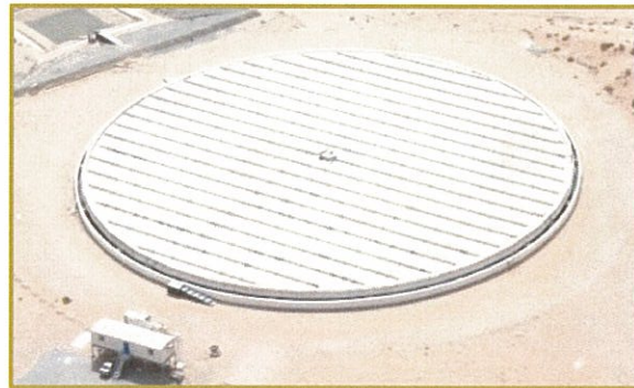
Precision solar tracking platform (5000 m2)
